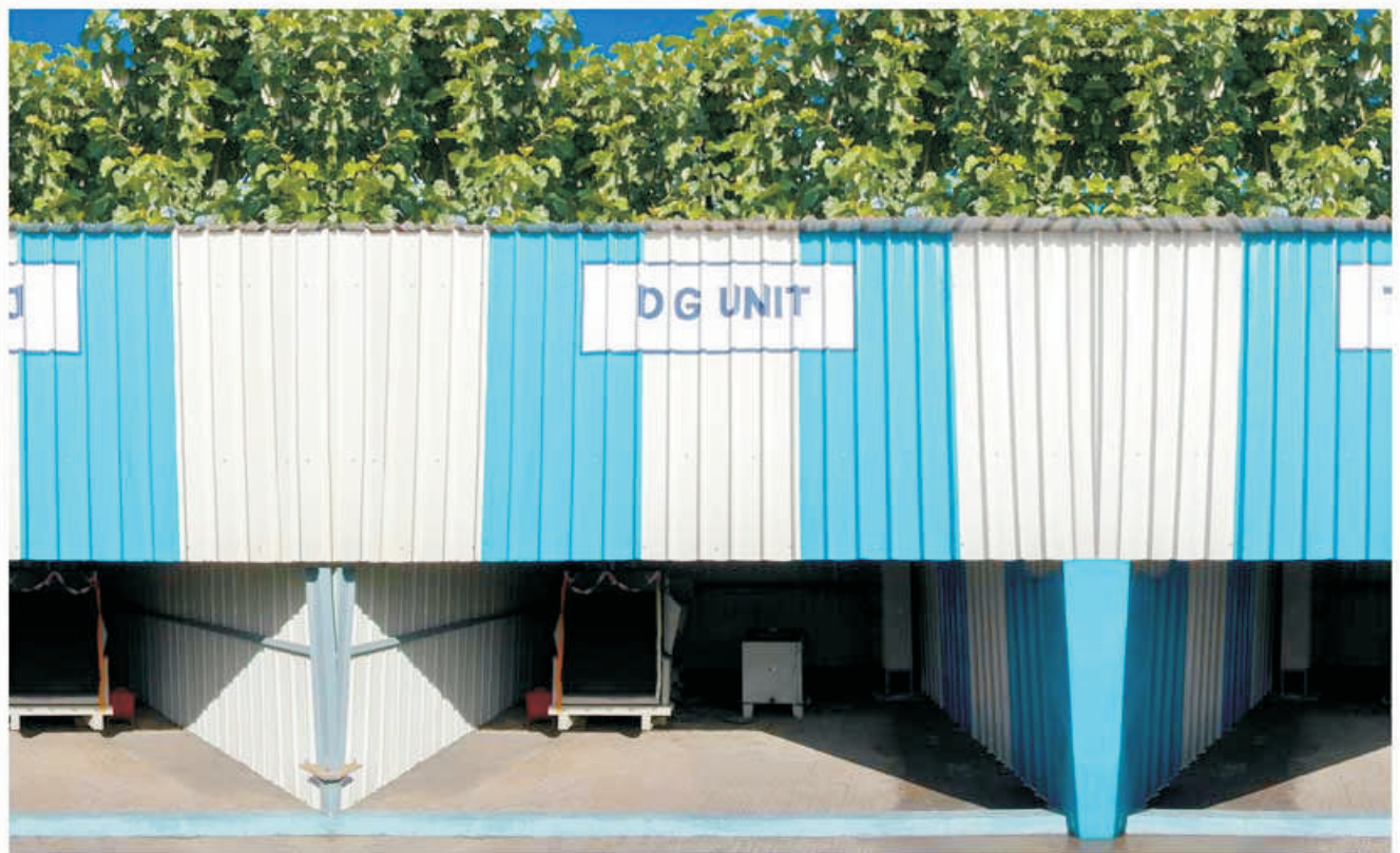
DG UNIT - 183 KW
